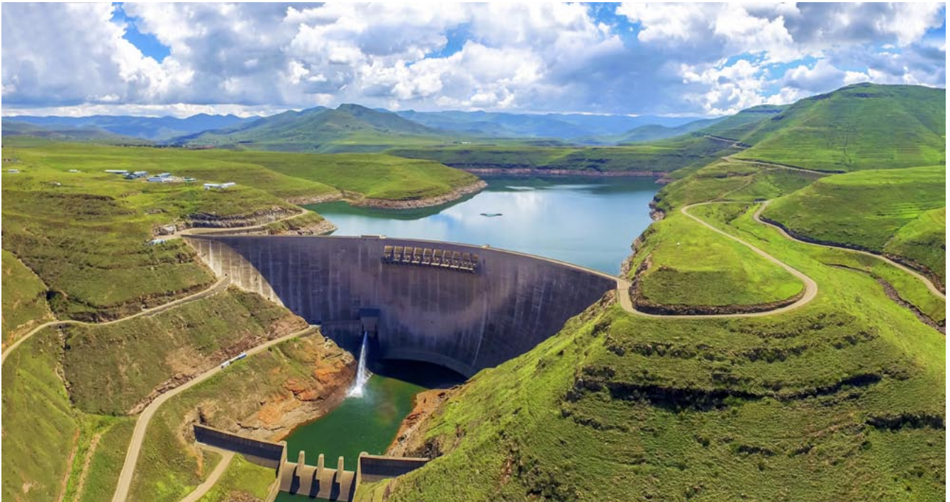
Lesotho's Katse Dam on the Malibamat'so River - centre-piece of the Lesotho Hlhighlands Water Project
