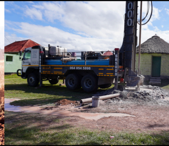
EASTERN CAPE MQHEKEZWEZI | BOREHOLE
