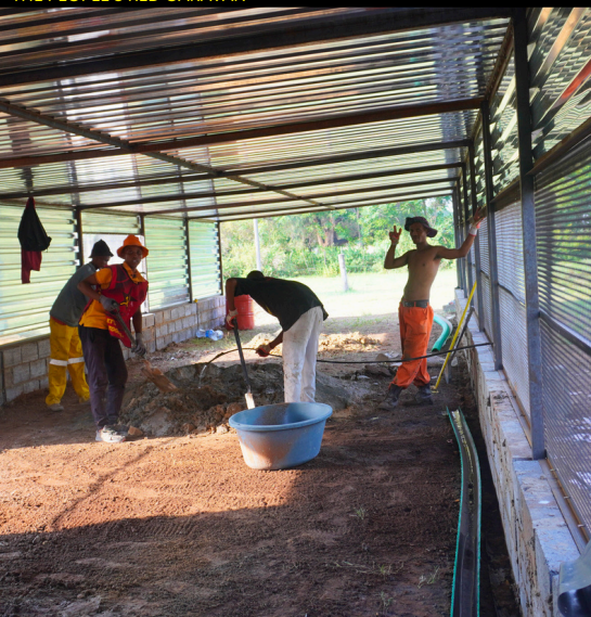
NORTHERN CAPE GANSPAN | CHICKEN COOP CONSTRUCTION
